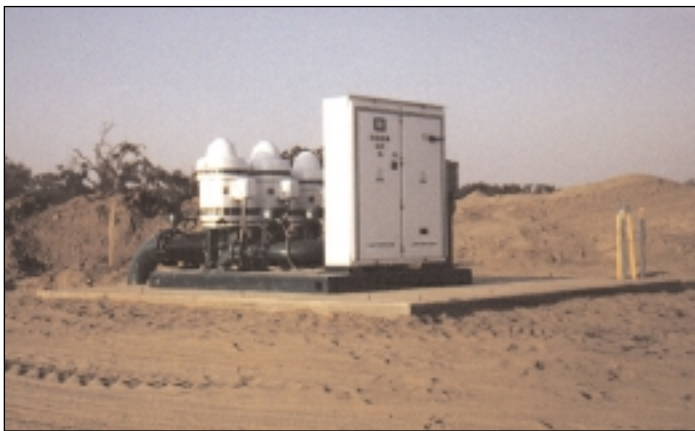
Dove Valley Phoenix, AZ 2200 GPM EBV Pressure Regulation Electronic Soft Starting
