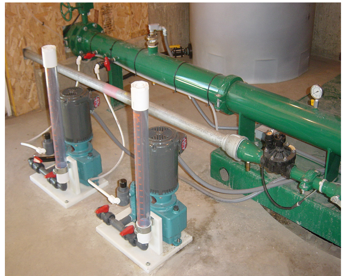
Typical installation of a EZ Feed Model 2-80
