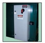
NEMA 4 service rated, main disconnect with lightning surge protection to safeguard station electronic components from power surge. (optional vandal resistant alarm light to provide external indication of pump station fault)
